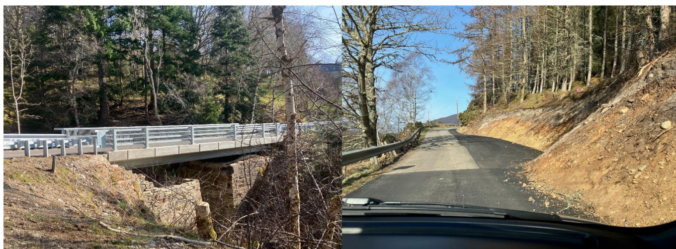
Figure 7: The U1991 was previously classed as an Excluded Route according to the Agreed Route Maps. The upgraded bridge and remediated landslip allow for a much shorter and safer route for both locals and timber lorries.
