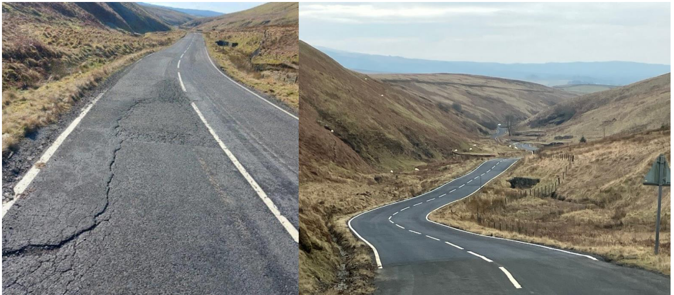
Figure 5: The B709 before improvements showing cracking and crazing defects indicating partial or total failure of underlying layers supporting the road surface leading to potholes and edge failures, and the improved road which will enable more sustainable timber transport for years to come.
