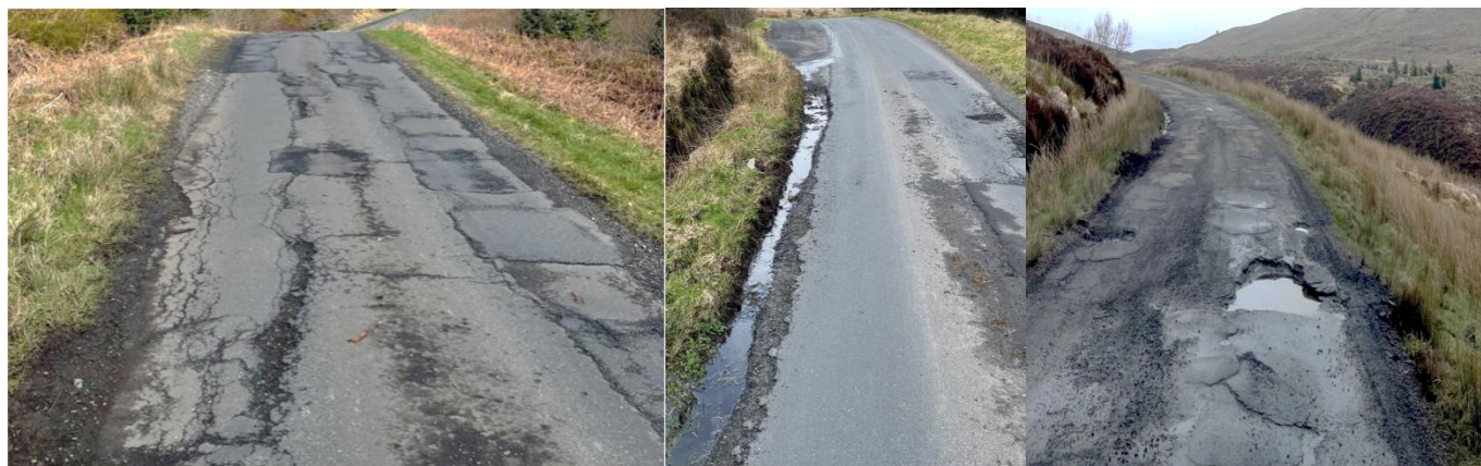
Figure 6: High altitude roads such as the C1 in Ayrshire are much more exposed to severe weather like frosts and pooling water leading to accelerated damage. Some sections of had deteriorated to a point where they were becoming unsafe with weak edges, potholes and pooling water.
