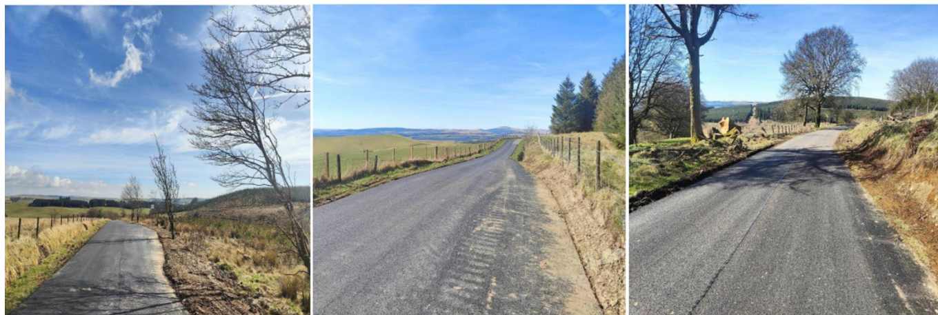
Figure 8: The upgraded and widened running surface and formalised passing places on the the C102a at Boreland improved journey times and safety for all road users.
